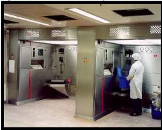
Flow booths can be equipped with partial or full screens with glove ports, potentially offering a further level of containment. These screens can be divided in:
